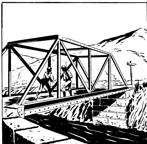
OVERHEAD STEEL BRIDGES
